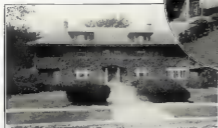
Typical of the homes that grace Oak Park, is this lovely place on Euclid Ave. In the circle above are shown six shops on Marian Street heated by Oil-O-Matic.
